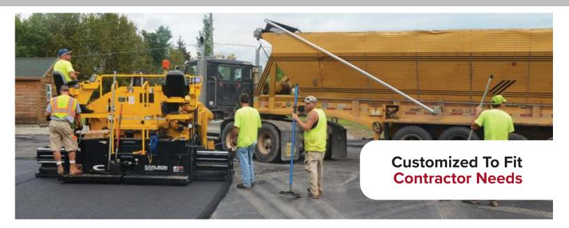
Representing the new standard for included features that enhance operator comfort, paving performance and mat quality, the CP130 is able to be customized further to the needs of any contractor. From wide pave attachments to grade and slope automation systems, the CP130 can be ordered with the options or added at any time.
